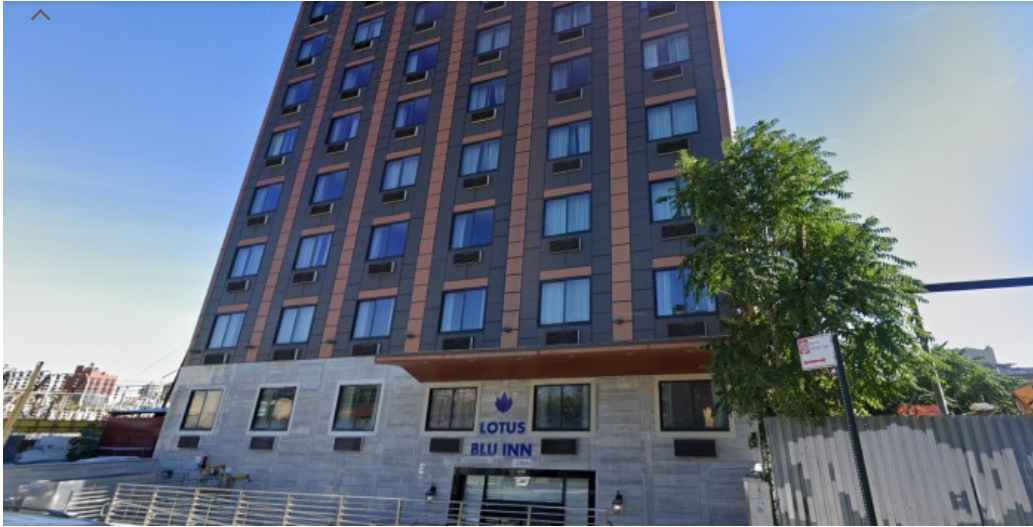
23-07 39th Avenue (Credit - Google)
